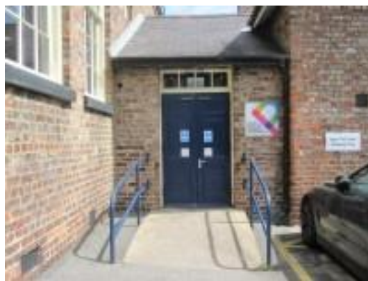
Image: Ramp and support handles leading to double doors
